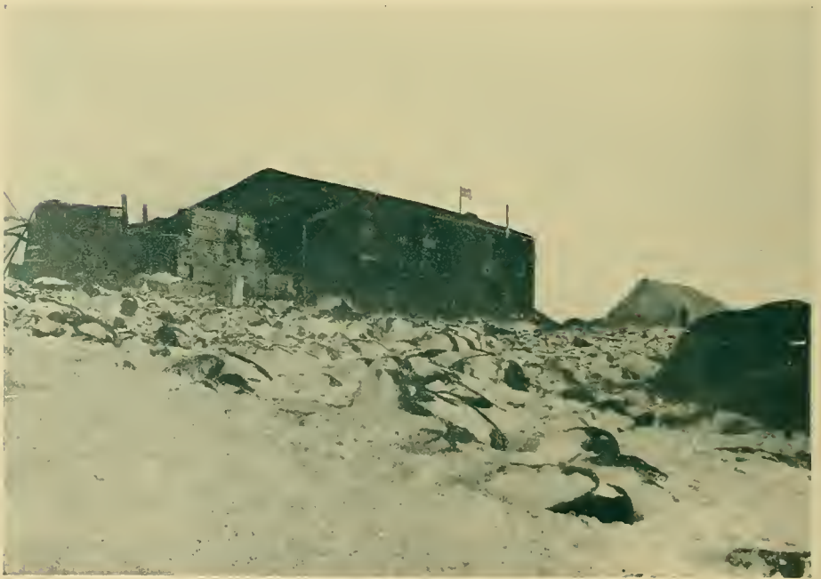
"ON SEPT. 24TH, THE HOUSE WAS COMPLETED"
